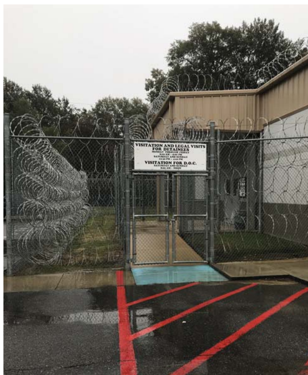
Richwood Correctional Center, Visitor's Entrance
